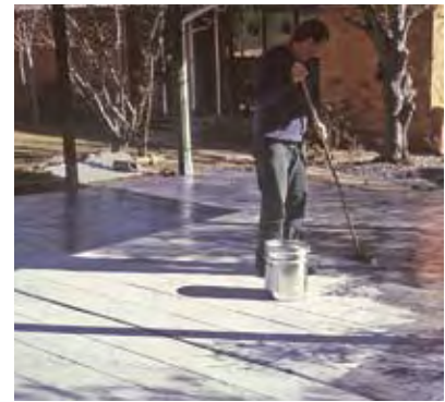
Figure 9 Sealing the surface to prevent staining
