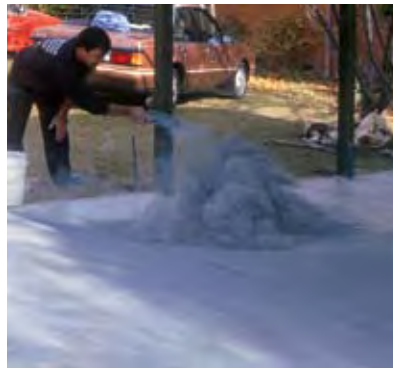
Figure 5 Dry-shake topping being applied
