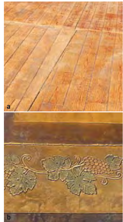
Figure 22 Finishes requiring reproduction of fine details stamped into a mortar topping [a] Timber pattern [b] Artistic pattern – colour from chemical staining
