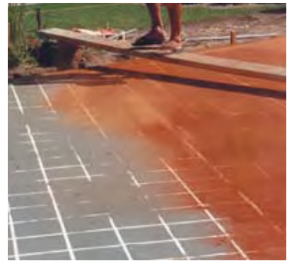
Figure 25 Access to all parts of the surface should be made available to ensure uniform application and trowelling of dry-shake topping (with permission from Concrete Technologies)
