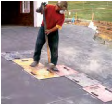
Figure 29 Stamping with textured rubber mats – slate texture aligned with joints
