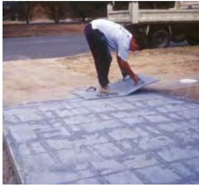
Figure 30 Completing edges
