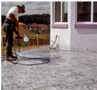
Figure 35 Removing the release agent with high-pressure water
