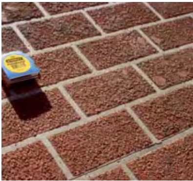
Figure 19 Various surface textures can be applied to improve slip/skid resistance
