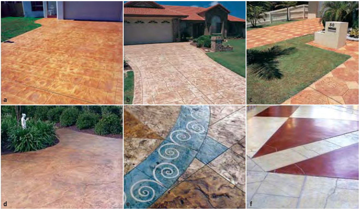
Figure 20 Some of the many stamped patterns and textures available [a] Random blue stone (with permission from Concrete Colour Systems) [b] Flagstone (with permission from Concrete Technologies) [c] Large diamond tile (with permission from Concrete Technologies) [d] Seamless (with permission from Concrete Technologies) [e] Rock texture [f] Slate texture
