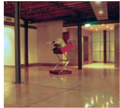
Figure 3 Floor placed in chequerboard pattern to conceal colour variations between concrete batches
