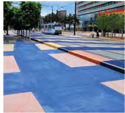
Figure 13 Worn areas apparent on surface coating
