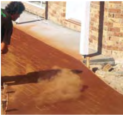
Figure 17 Applying coloured surface hardener over stencil
