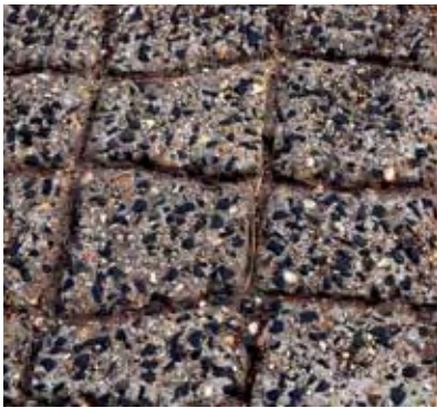
Figure 23 Stamped finish with aggregates exposed
