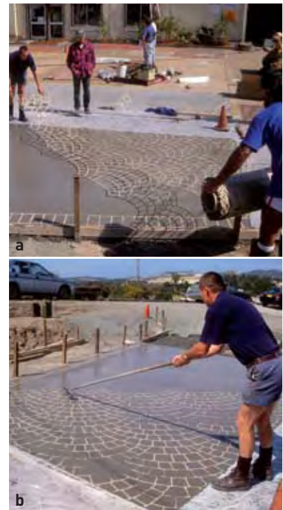
Figure 16 Placing and embedding the stencil into the 'wet' concrete
