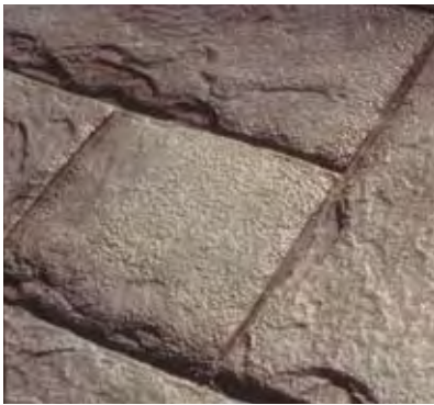
Figure 26 Surface textured prior to stamping to provide slip resistance
