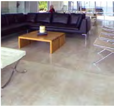
Figure 1 Off-white cement used in concrete topping
