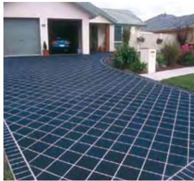
Figure 8 Dark colours may require three applications of colour hardener to ensure consistent colour
