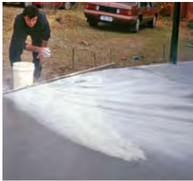
Figure 27 Applying release agent to surface
