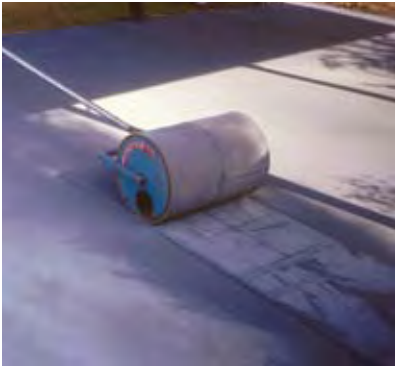
Figure 32 Stamping with a purpose-made roller
