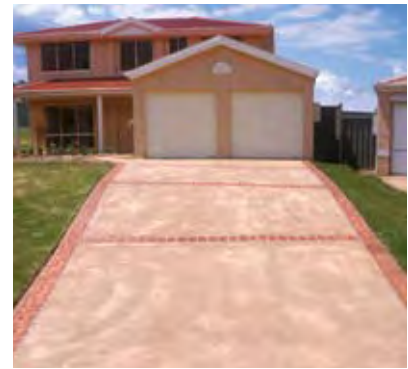
Figure 6 Dry-shake toppings used to provide surface colour to plain concrete
