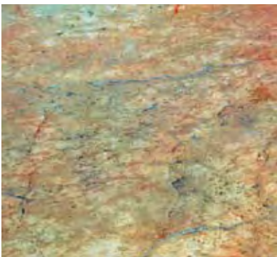
Figure 34 Seamless stamping mats used to produce continuous rock-like textures
