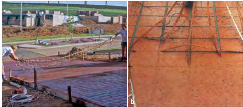
Figure 18 Stencil being removed ((b) with permission from Concrete Technologies)
