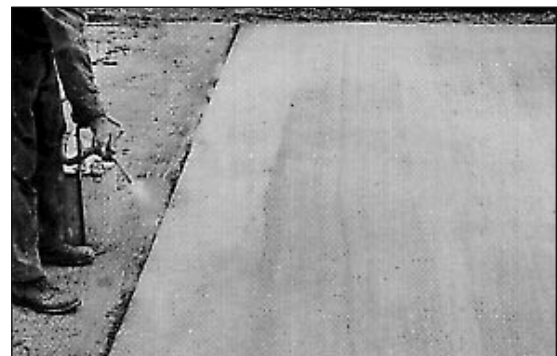
Figure 5: Spray application of curing compound
