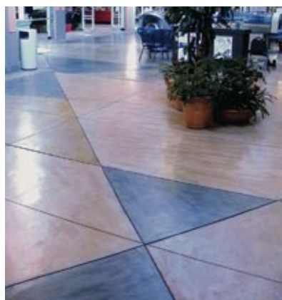
Figure 49 Joints used to create patterns in the floor and to separate colours/finishes
