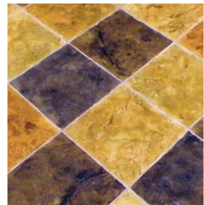
Figure 13 Slate texture in thin topping. Coloured using chemical stains
