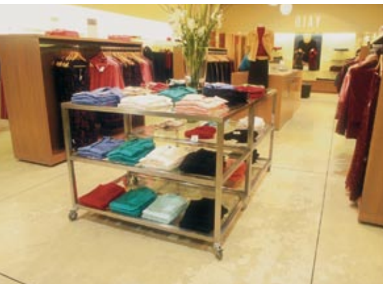
Figure 33 Surface sealer has worn and requires reapplication to restore surface lustre. Figure 4 shows the floor when first sealed.
