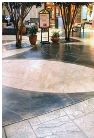
Figure 50 Random stone patterns have been formed by cutting joints in the thin 10-mm-thick topping to existing slab. Pattern can be used to conceal any random cracking in the existing slab
