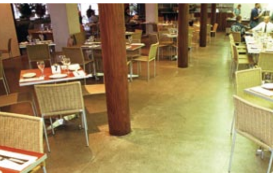
Figure 47 Joints (on column lines) formed with brass strips
