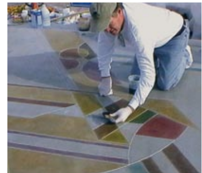
Figure 17 Application of stain by brush is generally suitable only for small areas.
