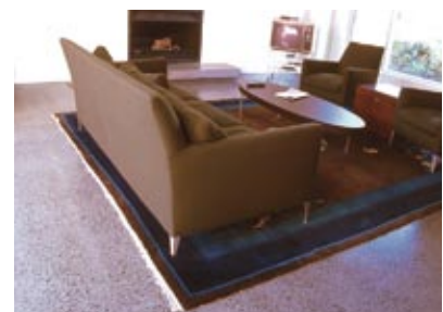
Figure 42 Sand streaks in the finish may be subtle and add to the character of the floor
