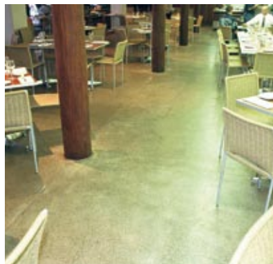
Figure 31 Regular cleaning will maintain the finish even in high traffic areas or those subject to frequent contamination
