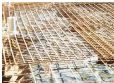
Figure 44 SL81 mesh used to control shrinkage cracking in polished section of residential floor slab.
