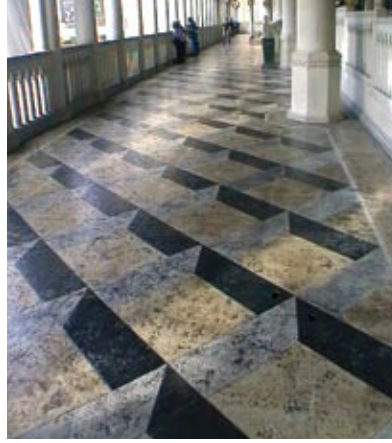
Figure 14 Chemically stained concrete floor providing three-dimensional appearance
