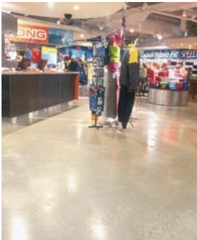
Figure 52 Existing post-tensioned slab lightly ground and left exposed. Surface sealed to provide high quality 'polished' appearance.
