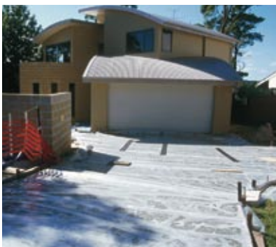
Figure 43 Clear plastic sheeting used for external applications
