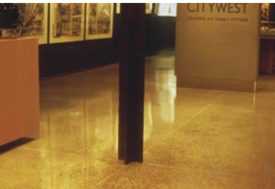
Figure 46 Saw cut joints in line with columns
